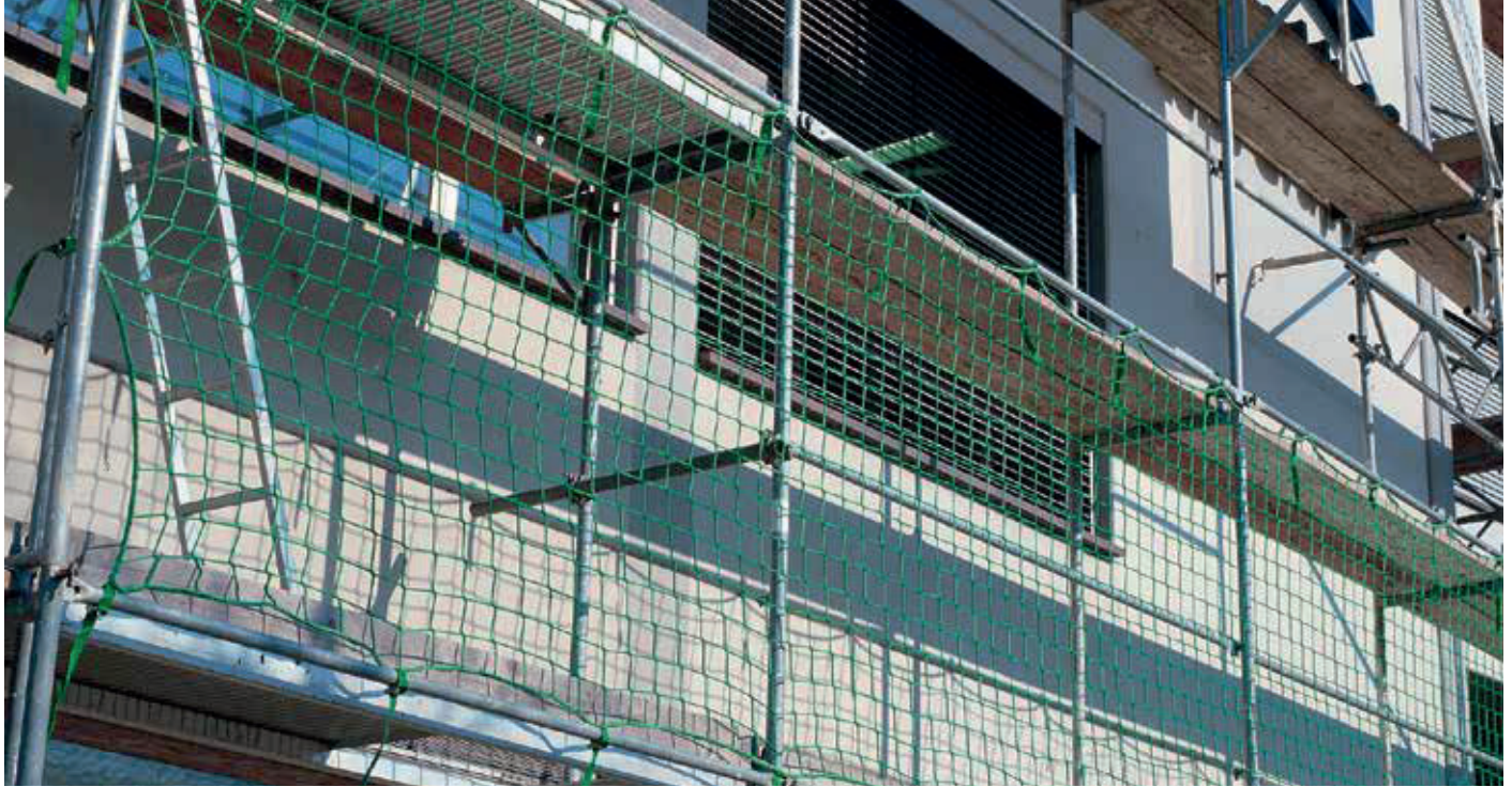
Brick guardrail net, mesh size 100 mm.
