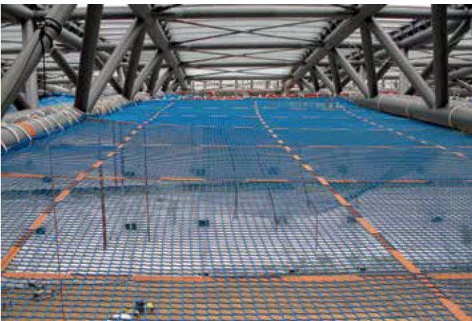
A personal safety rope is also required for the application illustrated above.
